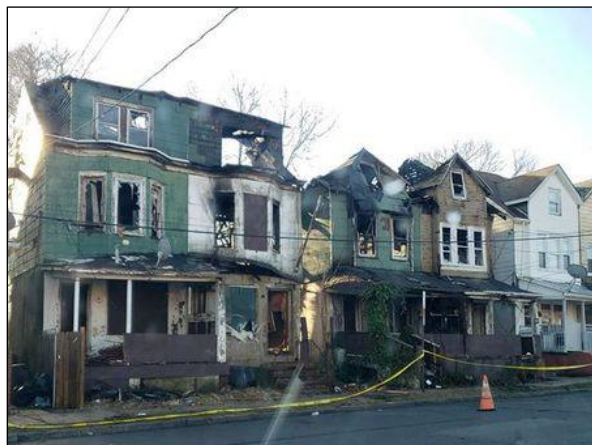
FIGURE 5-16: Multiple Closely Spaced Wood Frame Dwellings Damaged by Fire
