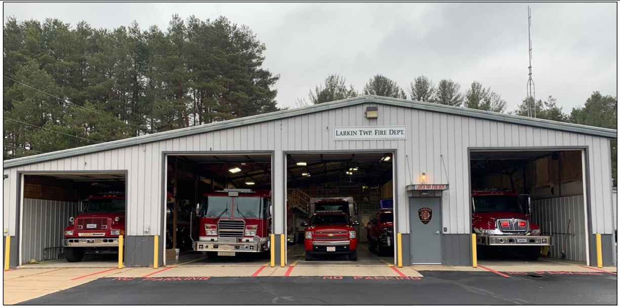
FIGURE 3-7: Larkin Township Fire Department Fire Station
